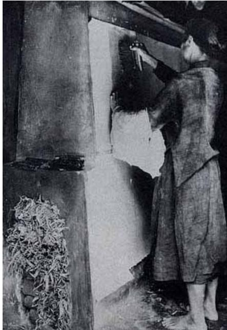
The sheets would be applied to the entire oven wall. As they dried rapidly, they could be detached after a short time and the space left available for the next sheets. Sheets would also be dried on unheated walls. This would
